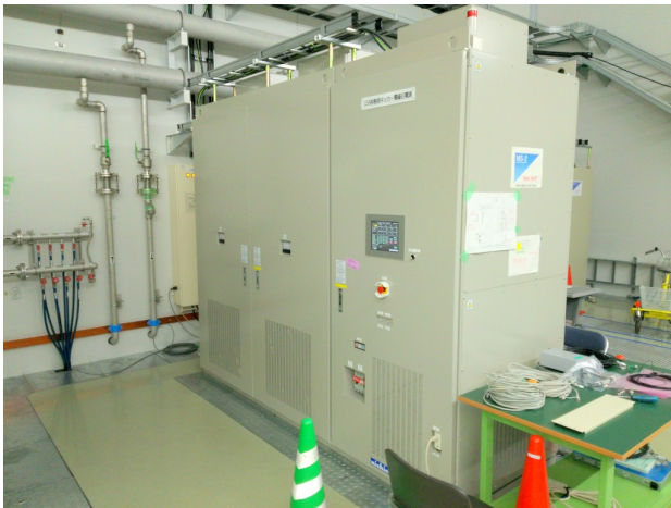
Power supply (60 Hz, 1 kV-299 A)
